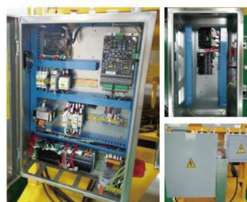
·Escalator control cabinet
